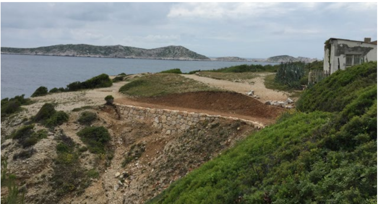
Creation of a retainer wall in Marseilleveyre before / after (top / bottom)
