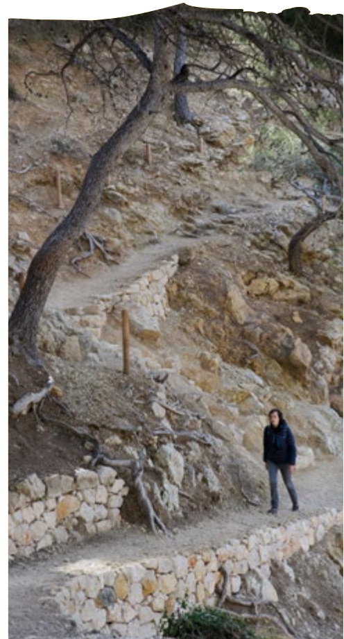
Heavily eroded trail before (left) and after (right) levelling work and the completion of installations (retaining walls) in Sugiton
