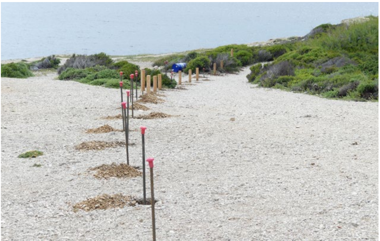
Post and wire installation in Marseilleveyre
