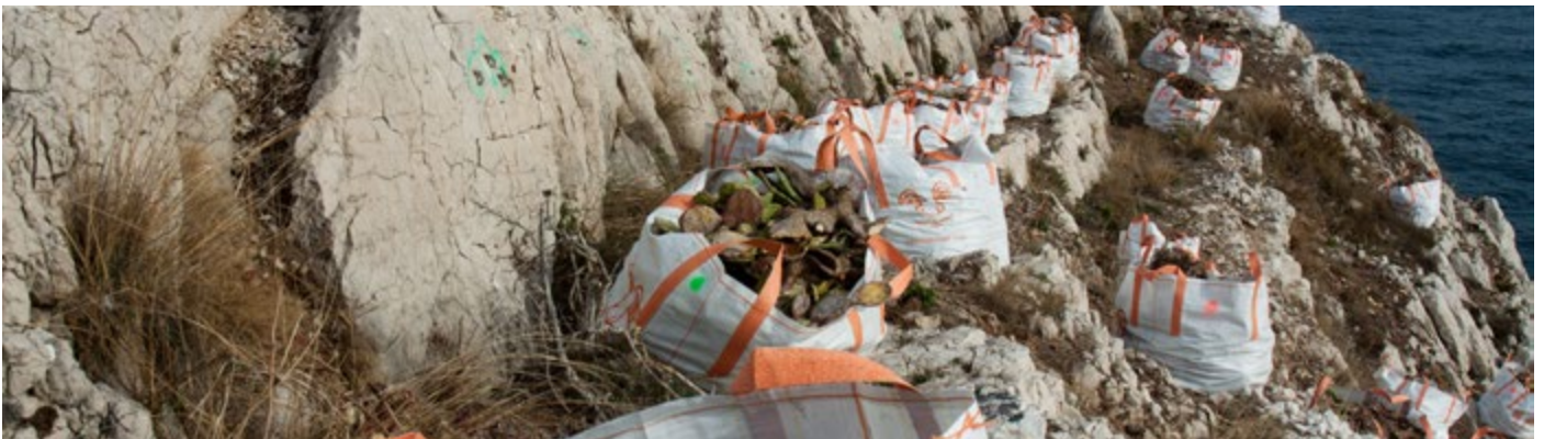
Slopes at Hôpital Caroline before/after the uprooting operation
