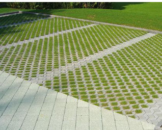
Surfaces semi-ouvertes Ratio = 0.5
